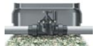
Coupling nuts are threaded onto the inlet and outlet of the valve
