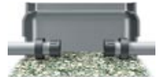
Fittings for the inlet/outlet of the valve are installed
