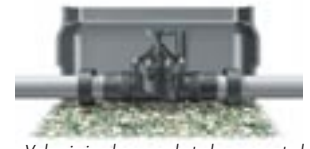
Valve is in place ready to be connected
